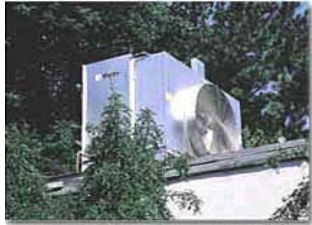
Figure 35: Fluid cooler cross flow with self-contained sump.
