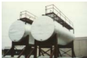
Figure 59: Horizontal tanks including concrete-lined tanks.
