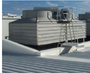
Figure 36: Cooling tower with self-contained sump.
