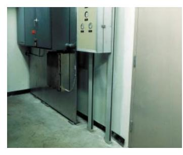
Figure 155: Two different ways to support control panels: using a metal plate attached to floor and ceiling with steel angles (left); using struts extending to floor and ceiling (right).
